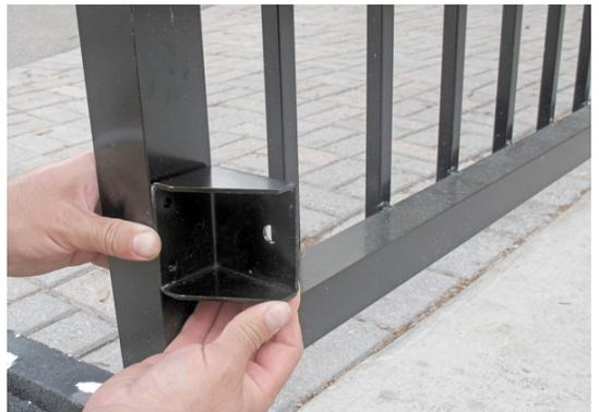
On one side of the gate lay the belt into the belt attachment bracket so the teeth of the belt mesh the teeth of the bracket.
