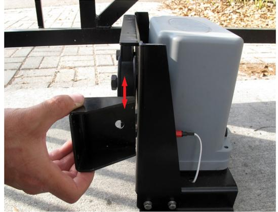
**Vertical position of gate bracket:** The hole in the gate bracket should be level with the top of the idler gears when mounted on the gate.
